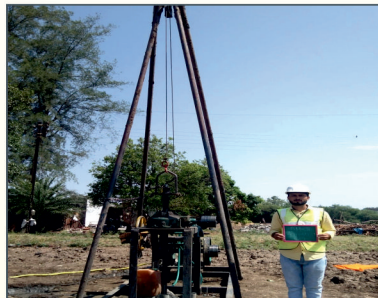
SOIL INVESTIGATION BY BORE HOLE METHOD
