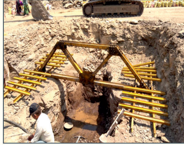
PLATE LOAD TEST BY TRUSS METHOD
