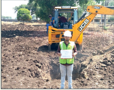
SOIL INVESTIGATION BY TRIAL PIT METHOD
