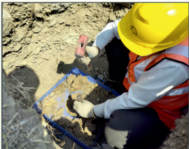
FIELD DENSITY BY SAND REPLACEMENT METHOD
