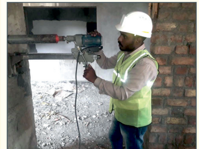
CONCRETE CORE CUTTING IN FIELD
